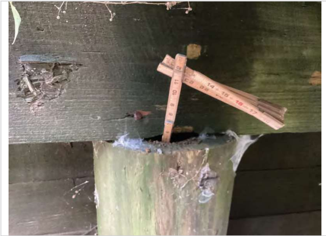
Top 1 pile G decay in top of pile
