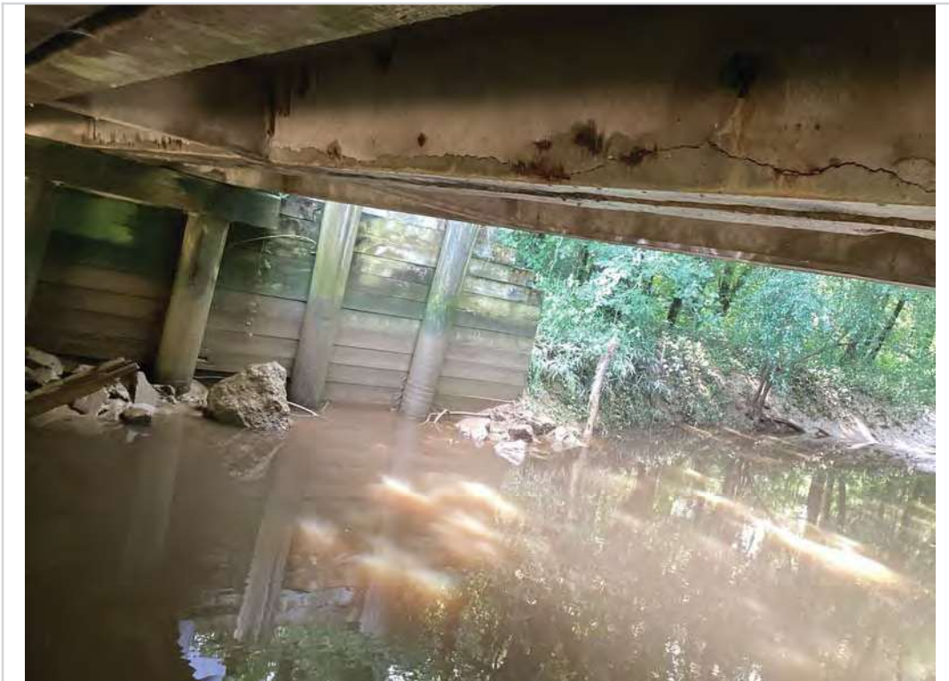
1/16" crack on slab G
