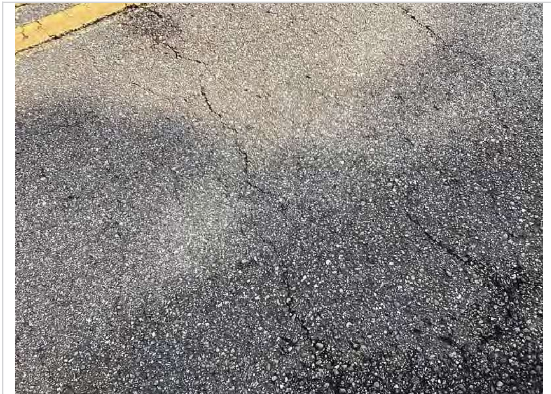
Wearing surface cracks
