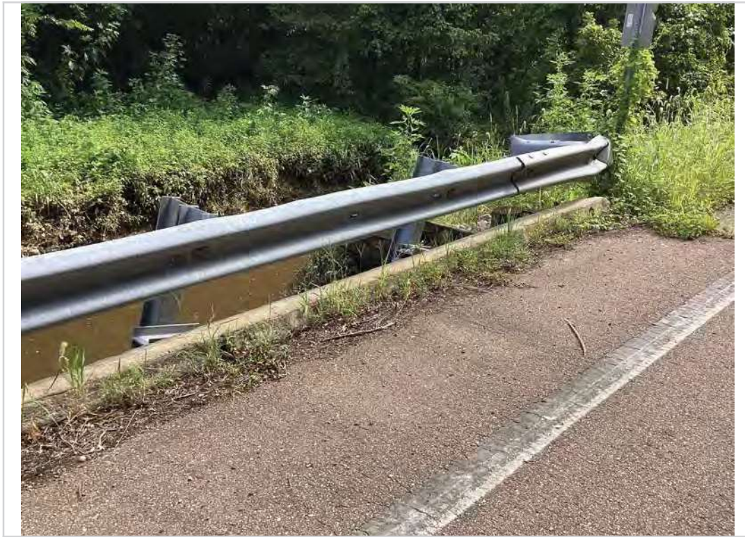
Left bridge rail damage
