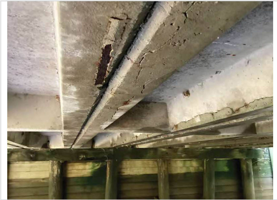
1/16" crack on slab D
