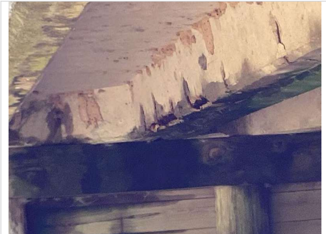
Spall to steel on slab A
