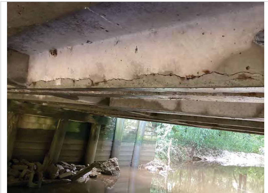
1/16" crack on slab D
