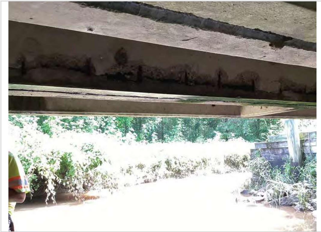
Spall to steel on slab B
